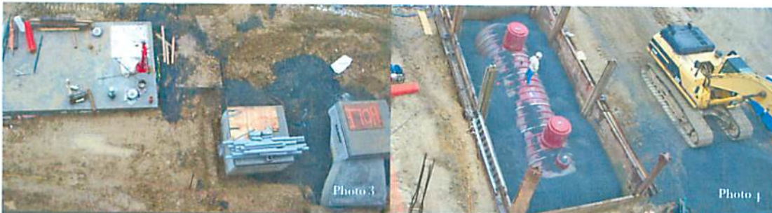
Photo 3: The neutralization tank and transformer vaults have been installed.
