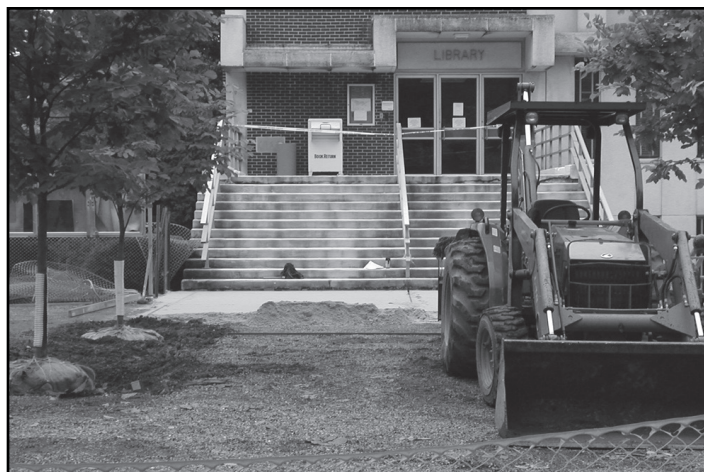
Construction begins on the library plaza.
